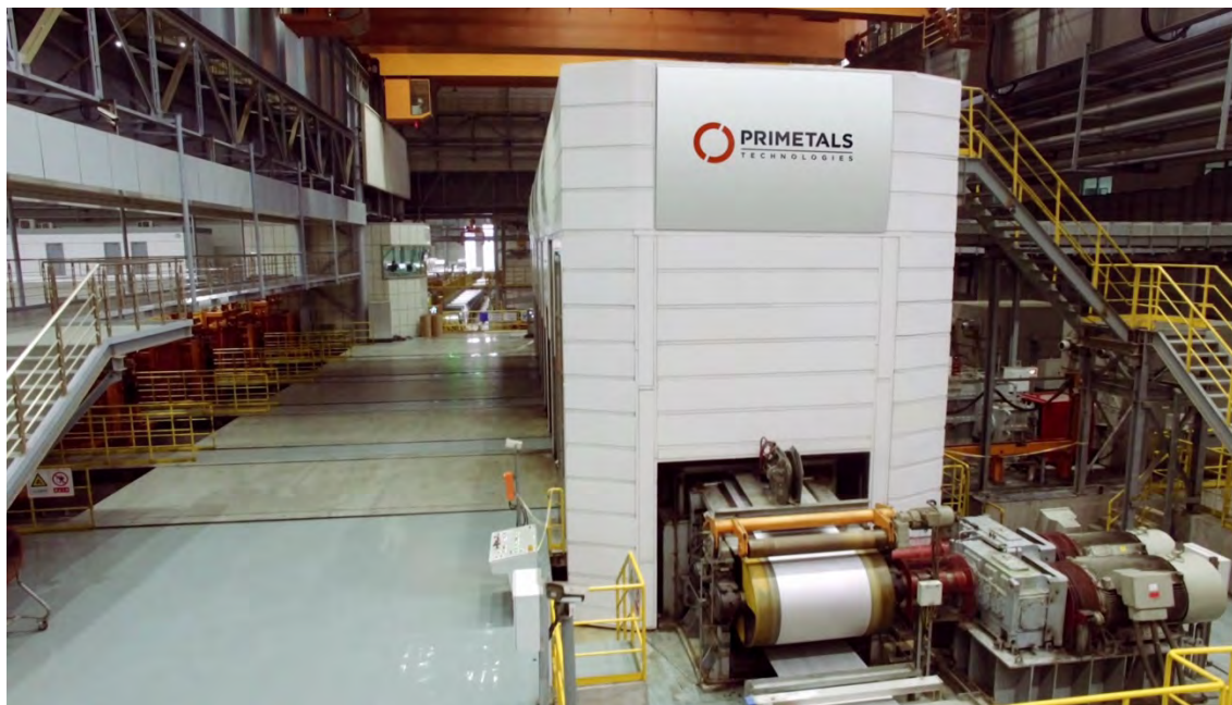
Cold rolling mill from Primetals Technologies at the Tangshan Iron and Steel Group Co. Ltd.
