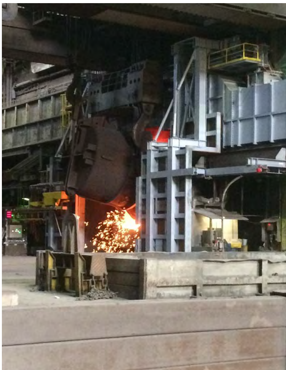
LD(BOF) converter from Primetals Technologies at ArcelorMittal Hochfeld in Germany
