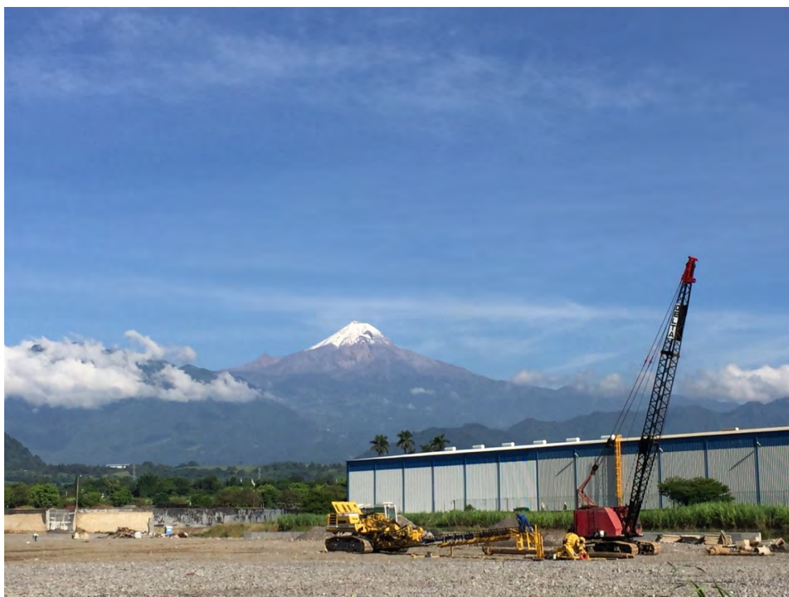
Excavation works for the first pier on Tyasa site for the combined galvanizing and color coating line
